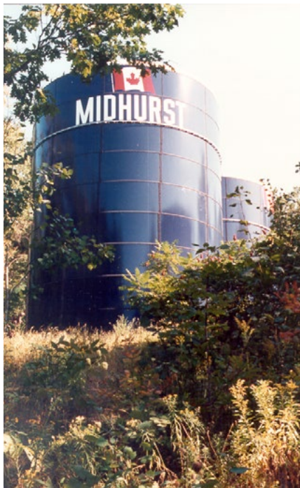
(Left) Greatario installed its first permanent glass coated tank in Midhurst in 1986. (Top right) Anodes installed on the glass fused to steel floor can be tested from the outside of the tank using a multi-meter +CSE per NACE requirements, while the tank is in service (bottom right).
